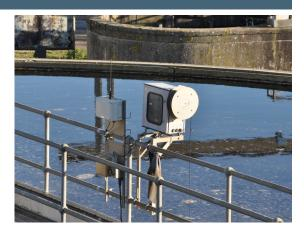
The ASLD2200 is a fully automatic sludge blanket level detector designed for the water and waste water industry. It utilises a servo-driven sensor which continally tracks the settled interface with the sensor at the very top of interface zone.
