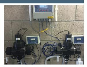
The ColTechw<sup>2</sup> Sensor has been specifically designed to monitor Apparent Colour in applications where a broad indication of the colour of the water is required. Organic materials such as Humic Acid or metals like Iron and Manganese dissolved in water will appear as an unacceptable yellow tinge. If discoloured water is allowed to enter the water supply network customers will quickly become aware of the problem.
